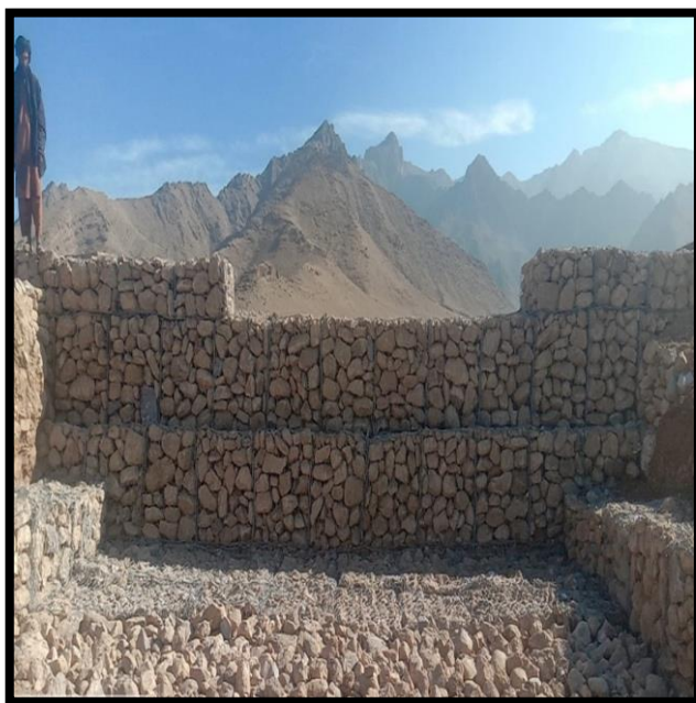
Pic5: CFW, Infrastructure project, Check Dame, OSRO/AFG/130/CHA project, Dehrawood district of Urozgan Province.
